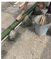
③汚れの清掃
